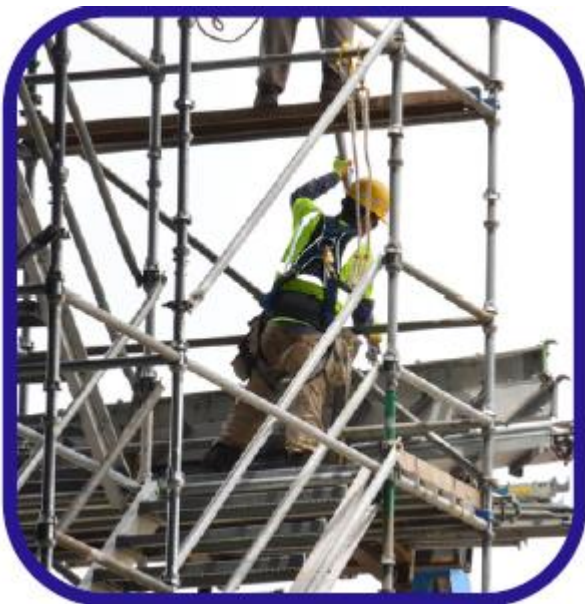
TAMANG SCAFFOLDING WORK
